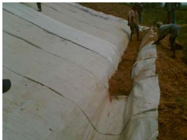
Fig. 6 : Trench at the base of the slope for anchoring of geotextiles by wrap-over method
