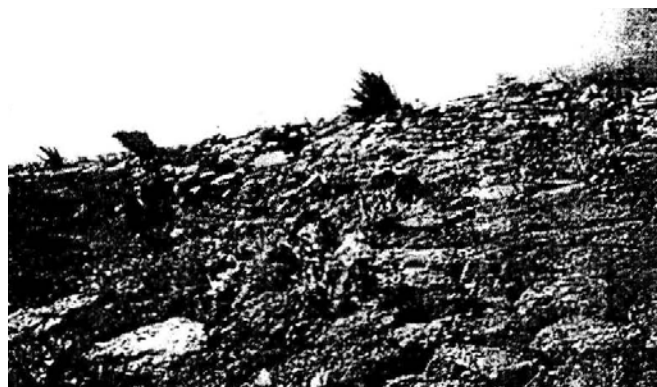
Fig. 2 : Stone pitching at in River Subamarekha
