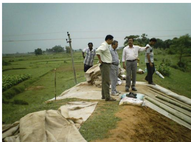
Fig. 1 : laying of fabric
