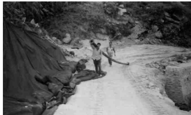
Photo 5 : Provision of subsurface drainage at the 'Camel back'
