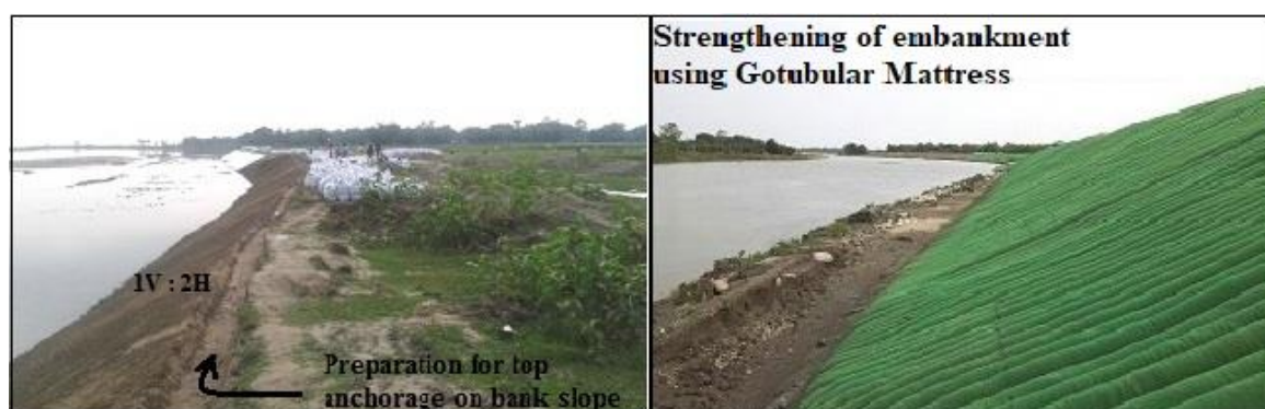
Fig. 7 : Strengthening of embankment using geotubular mattress (Tezpur W.R. Division, Assam)
