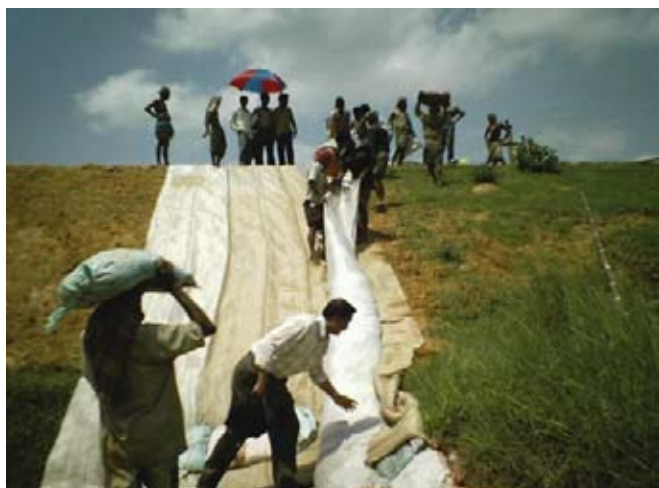
Fig. 7 : Geotextile-tubes being filled in for anchoring
