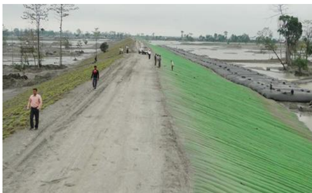
Fig. 9 : Geotubular mattress with scour apron at Matmara geo-dyke ( www.waterresources.assam.gov.in )
