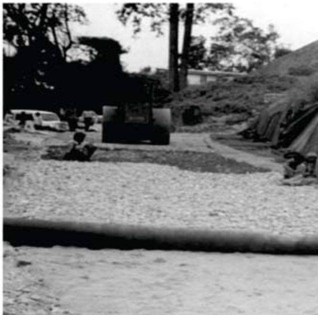
Photo 3 : Installation of GEOLON PP80 at Pango link
