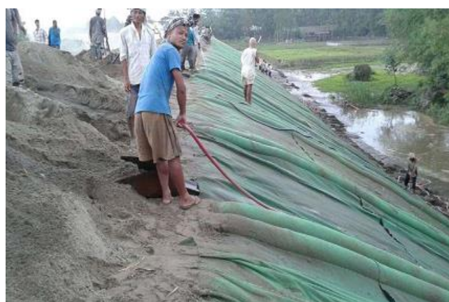
Fig. 2 : Geotubular mattress laid over prepared slope (North Lakhimpur, W.R. Division, Assam)
