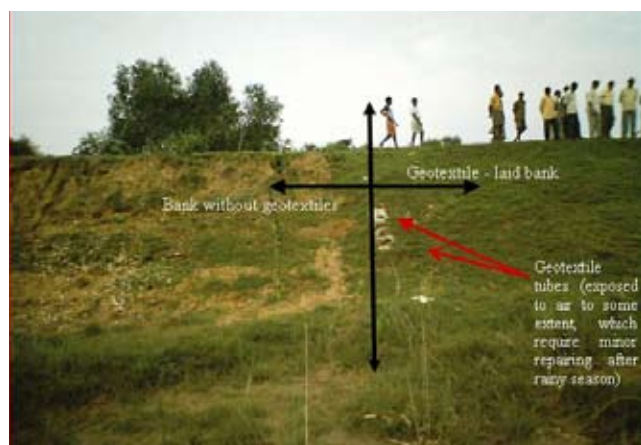
Fig. 17 : Photograph showing the difference between the parts of the river-bank constructed with geotextile and without geotextiles
