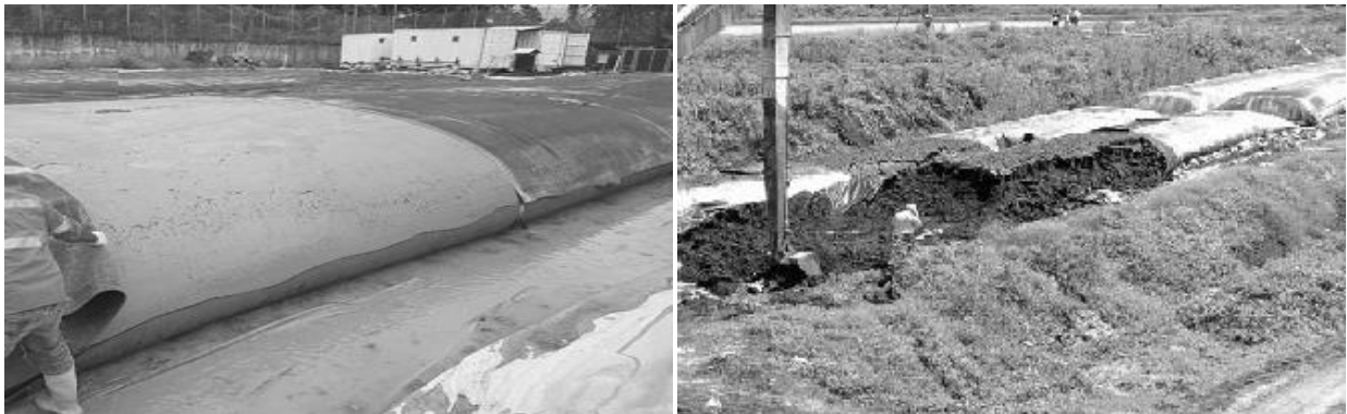
Fig. 13 : Disposal of solids from geotube container [12]
