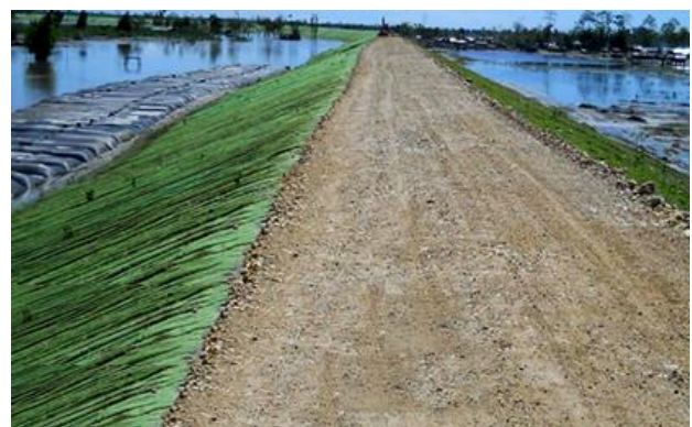
Fig. 9 : Geotubular mattress with scour apron at Matmara geo-dyke ( www.waterresources.assam.gov.in )
