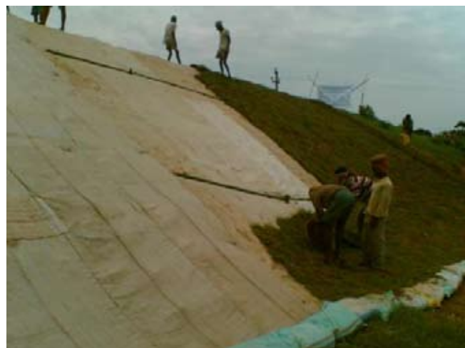
Fig. 8 : Covering geotextiles with grass-sods
