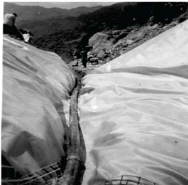
Photo 4 : Installation of perforated HDPE pipes at Pango link
